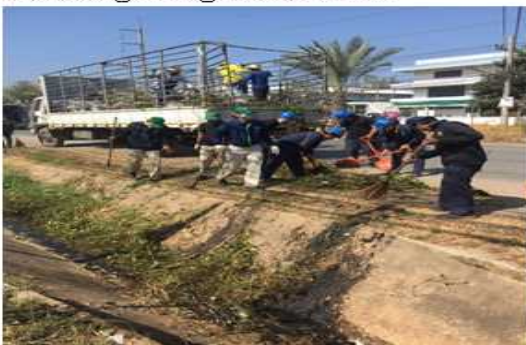
Cleaning rein gutter out side
